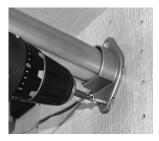
Using #8 (1 1/2") wood screws provided, secure one flange to wall stud on "non-wired" side of closet.
